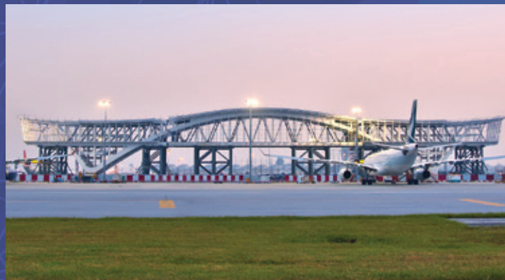
The three segments were delivered to the bridge site separately for assembly and construction.
