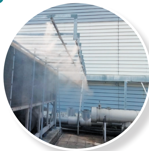
AAT has installed high-pressure tubes and fittings to enhance the energy performance of air-cooled chillers. 亞洲空運中心裝設了高壓管及裝置，藉以提高風冷式製冷設備的能源表現。
